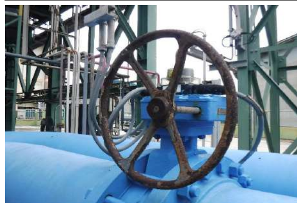
Pic. No. 12 Location : Butterfly valves
