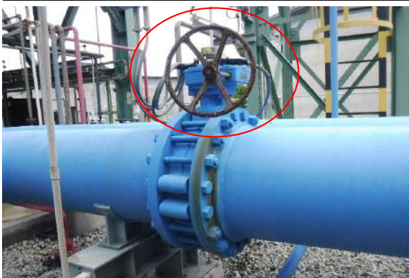
Pic. No. 11 Location : Butterfly valves
